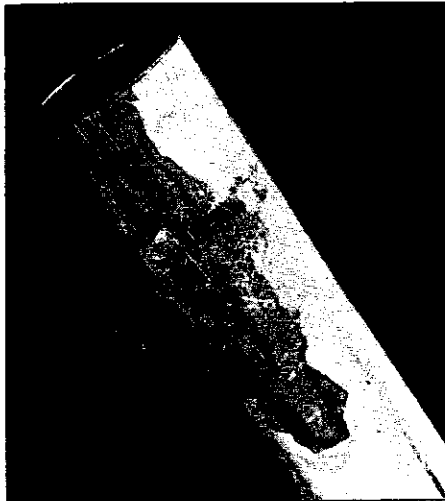
A recently disassembled, partially oxidized interior joint. The short, formerly telescoped tubing section looks much better than the adjoining element section that has been continually exposed to the elements. Nevertheless, it has oxidized.
