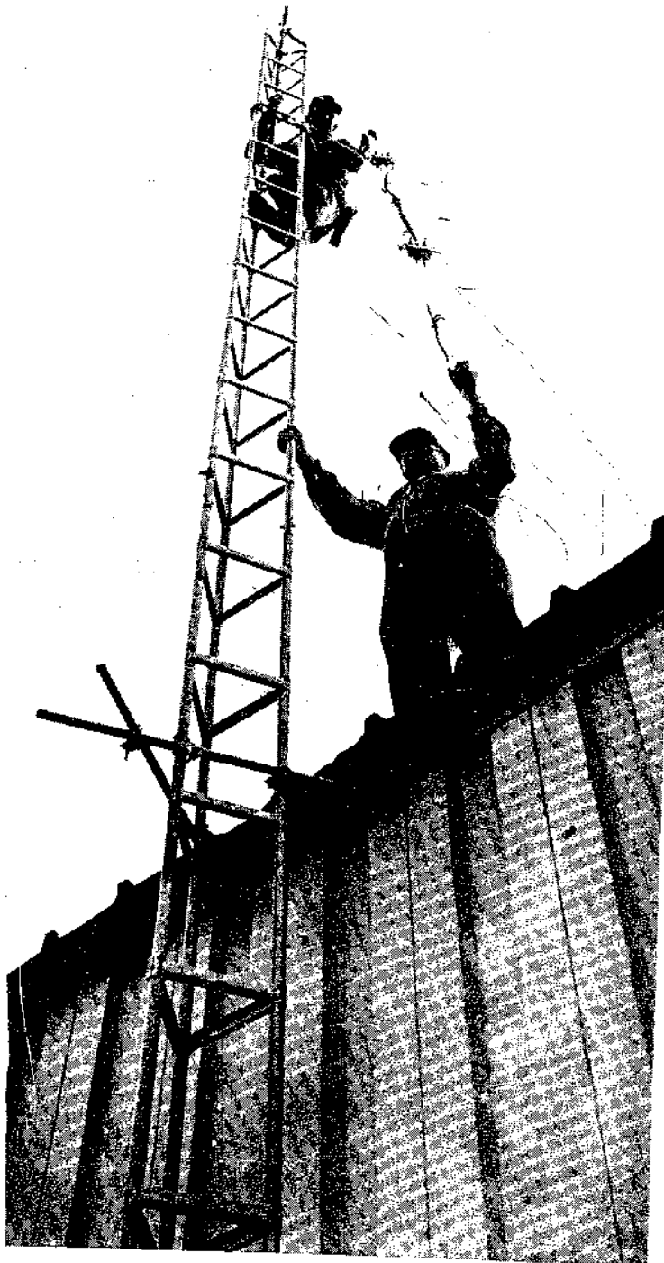
On Friday afternoon, Walter, VE3FFN, of Proton and Stan, Flesherton, climbed the tower at the Flesherton Arena and installed the antennas, used in the booth at the Split Rail Festival. The wind, rain and cold didn't help them in their task of setting up the system for the Club.
